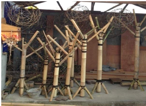
Gambar 6. Instalasi Tiying Canggah Wang (Foto: Eka Sutawan, 2013)
